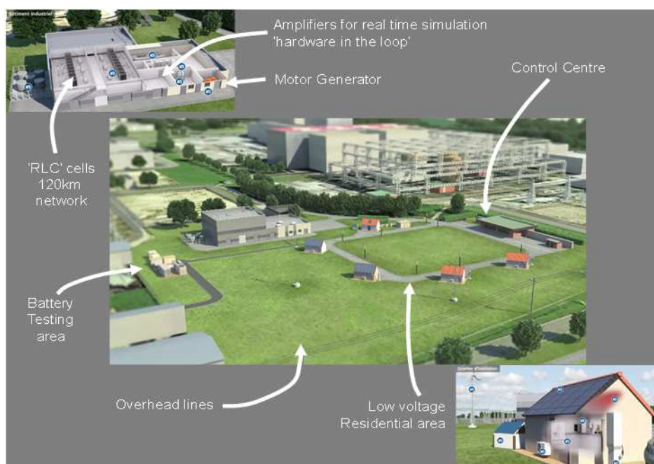
FIGURE 7: EDF CONCEPT GRID: A REAL NETWORK SPANNING FROM THE PRIMARY SUBSTATION UP TO THE METER AND END-CUSTOMER
