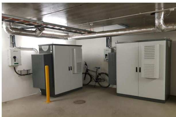
FIGURE 16. BATTERY ENERGY STORAGE SYSTEM AT THE OFFICE OF HELEN DSO. TWO BATTERY UNITS, 60 KW EACH. MODEL: TESVOLT, TS HV 70 OUTDOOR
