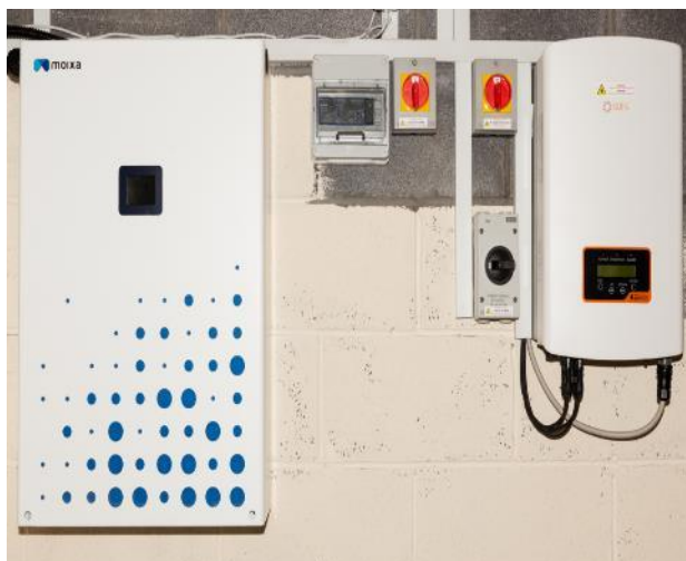
FIGURE 2. INSTALLED MOIXA BATTERY, SOLAR PV INVERTER AND OTHER ANCILLARY EQUIPMENT IN PARTICIPANT GARAGE
