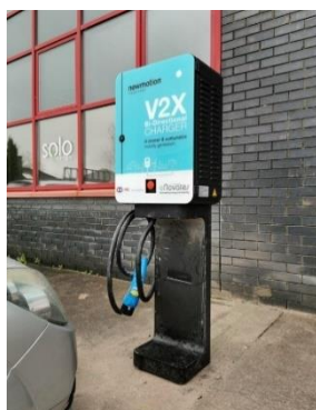
FIG. 10. V2G CHARGER INSTALLED AT SMS'S OFFICE
