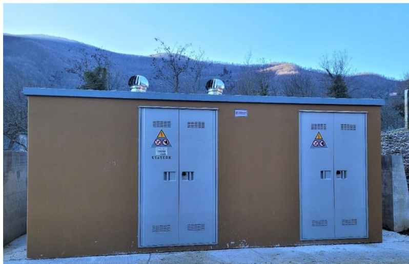
FIGURE 3-38 – SECONDARY SUBSTATION FEEDING STATCOMS.
