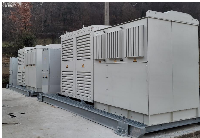
FIGURE 3-39 – VIEW ON THE TWO STATCOM MODULES INSTALLED IN QUARTO PRIMARY SUBSTATION.
