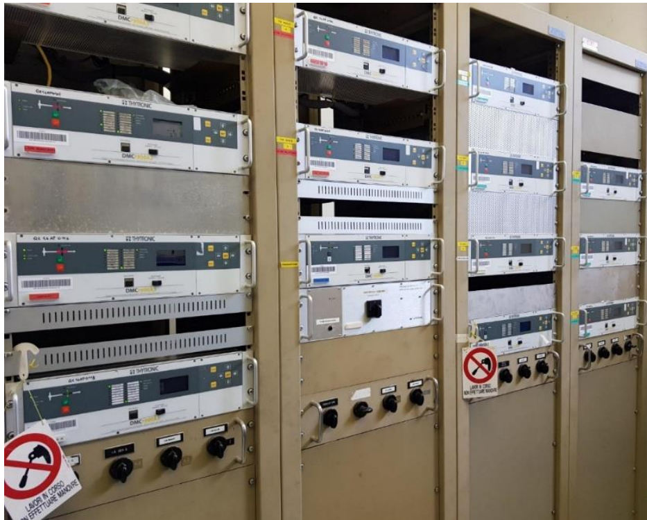
FIGURE 3-24 – VIEW OF THE FEEDER PROTECTIONS DV7203 PERFORMING FAULT DETECTION AND MEASUREMENTS COLLECTION.
