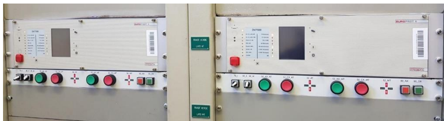
FIGURE 3-25 – VIEW OF THE INTEGRATED TRANSFORMER PROTECTIONS DV7500 PERFORMING FAULT DETECTION, MEASUREMENTS COLLECTION AND AUTOMATIC VOLTAGE REGULATION ON THE OLTCs OF HV/MV TRANSFORMERS.
